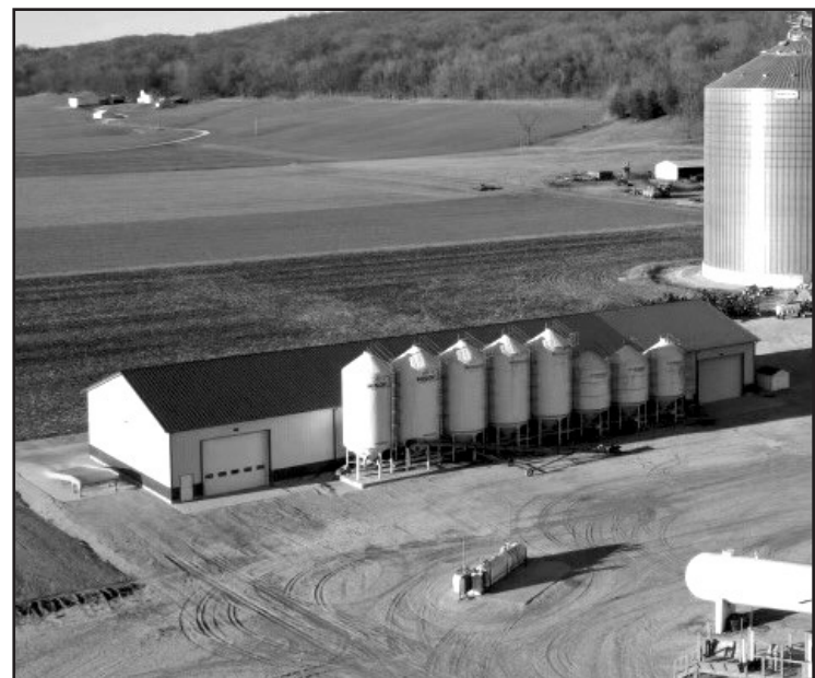
Chalfin Bridge Seed Shed Addition
